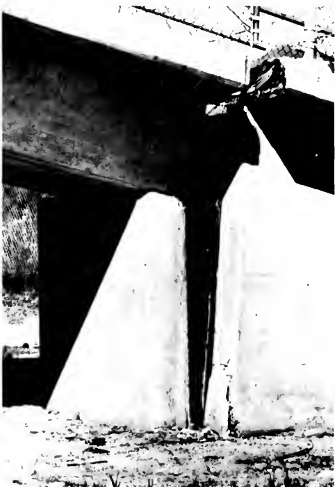
Photo 27. View of permanent support displacement, Tyler Street pedestrian overcrossing at Foothill Freeway [37].
